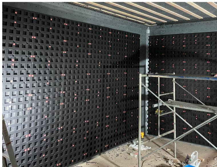
Hybrid EPP absorber base Fix unit Work with M4x50 screw
